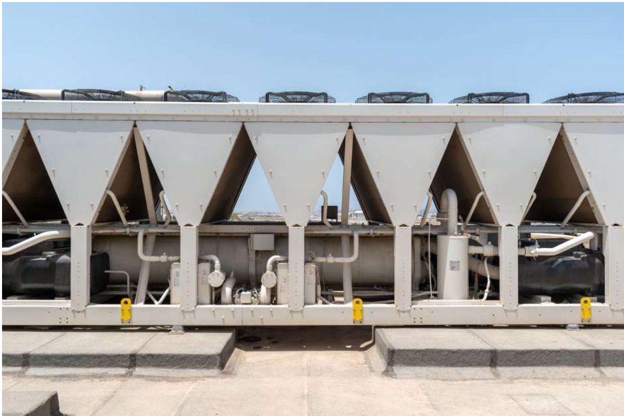
2023 Replacement of Chiller
