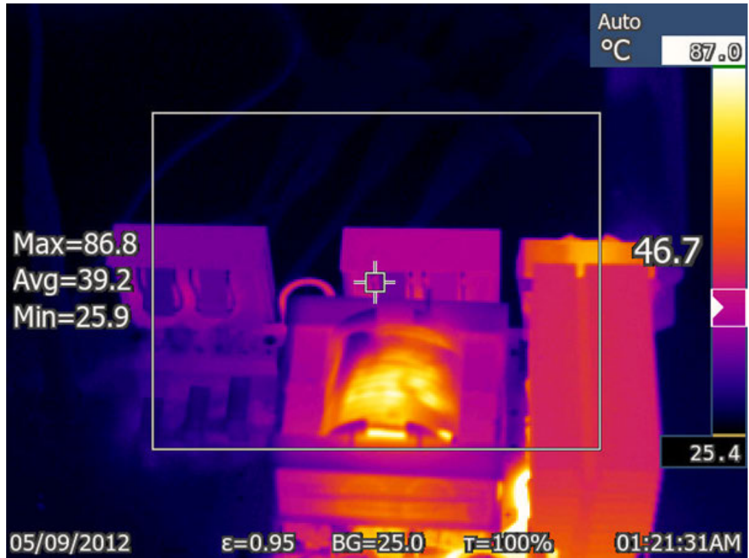
Figure 43. STDES-2KW5CH48V LLC thermal performance
